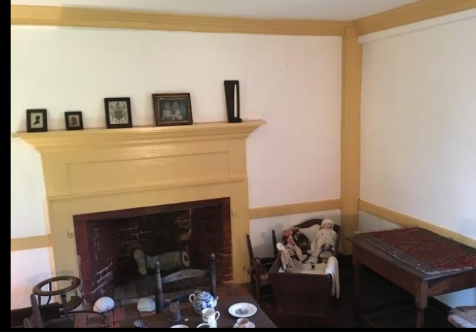
Room 205 NW Chamber NW-1. Cornice
